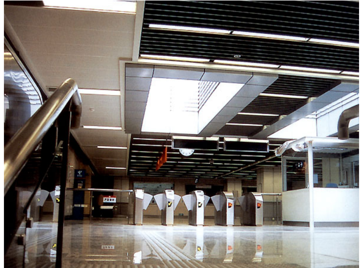
Figure 8. Subway Station Lighting
